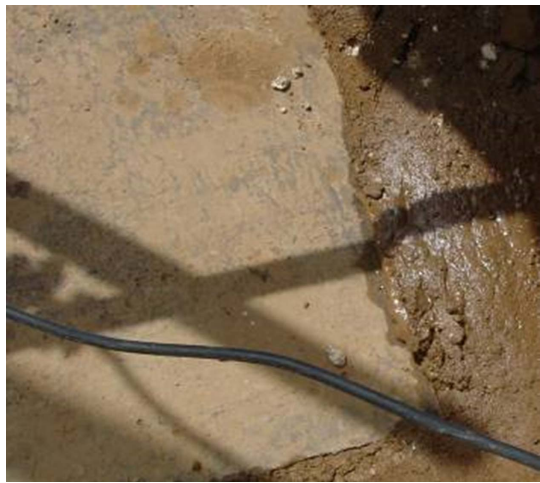
Fig. 6. Mud-pumping phenomenon of the liquefaction ground.
